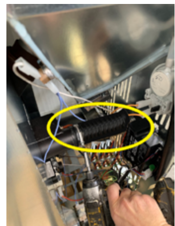
Fig. 60 - Raccorder le tuyau flexible
