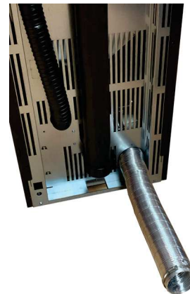
Fig. 79 - Raccorder le tuyau flexible
